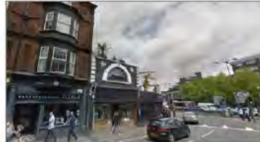
The existing Bridge Street elevation
