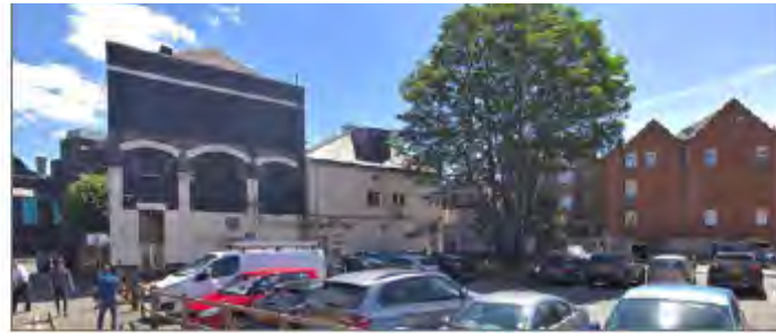
The existing rear view of the site
